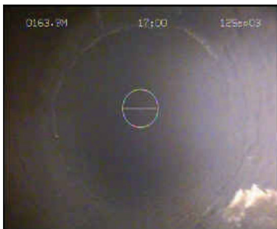
Figure 2 – Scale near bottom of Riser (2003)
